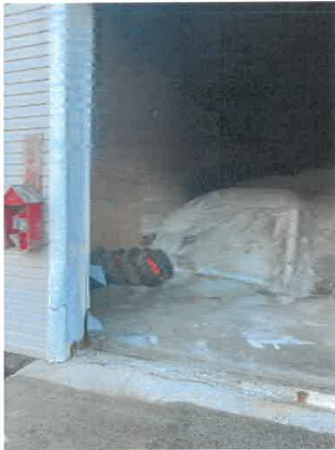
Photo 8. Inside of salt shed, left side.
