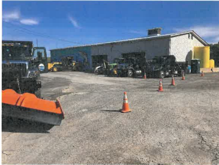
Photo 1. Milton's DPW Highway Garage. Salt shed bay is the one on the far right, and also seen are the two MgCl tanks (yellow), and the fuel tank (blue) next to them and behind the truck and port-o-let.
