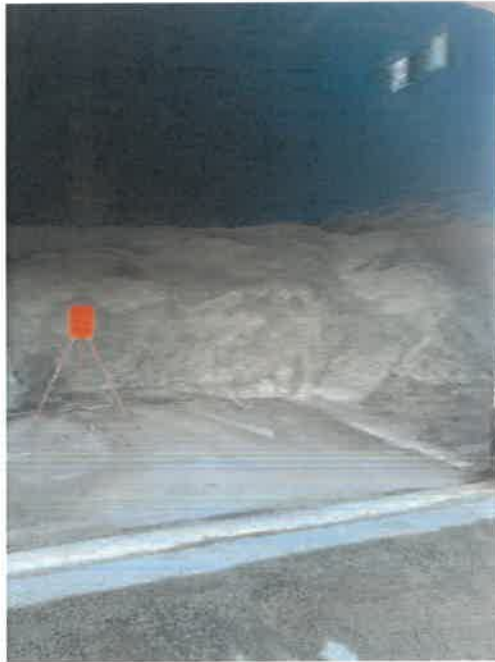
Photo 7. Inside the salt shed. Right side wall is bowed out due to weight of salt against it over time.
