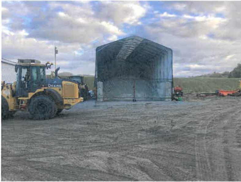
Photo 5. Temporary, supplemental salt shed constructed in fall of 2019. 200 ton capacity.
