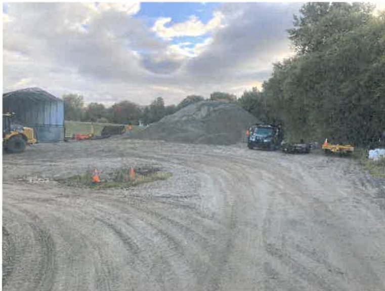
Photo 6. Temporary salt shed on the left, uncovered winter sand pile in the back.
