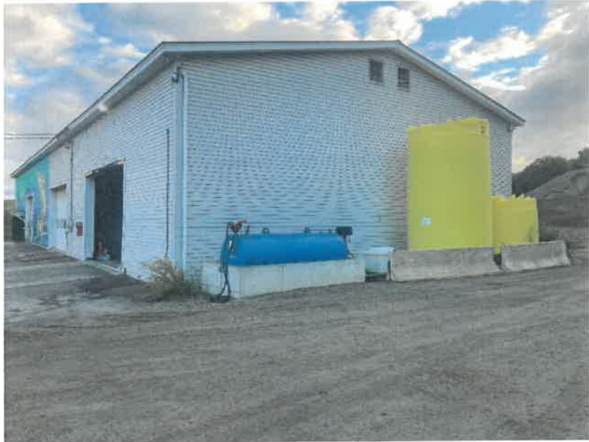
Photo 4. Fuel tank (blue), and MgCl tanks (yellow) behind jersey barriers.
